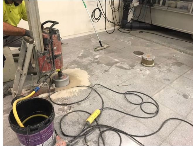
Drilling of the ground for the placement of water pumps
