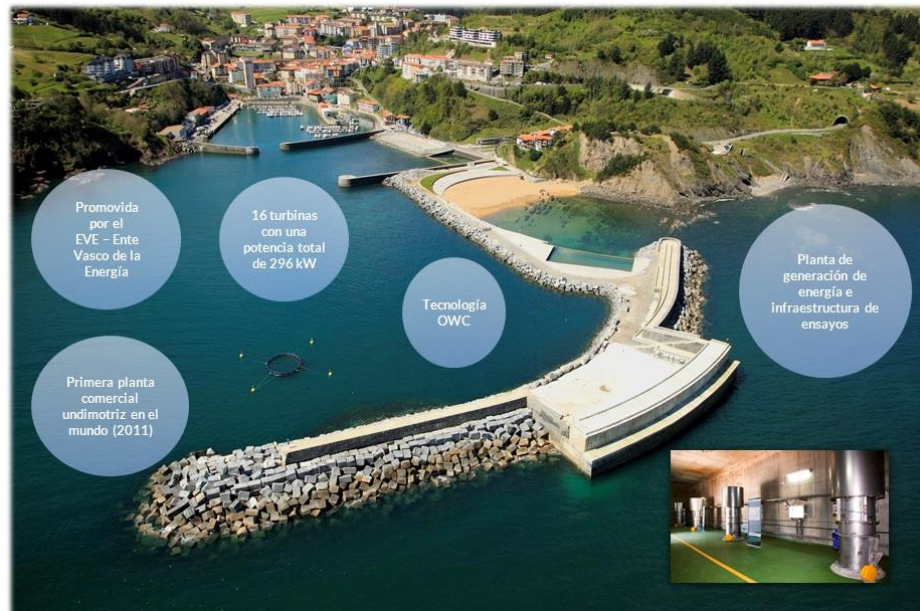
Mutriku Wave Power Plant
