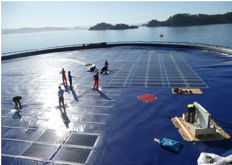
Installation of Ocean Sun's 100 kW offshore demonstrator in Kyrholmen (image: Ocean Sun)
